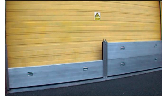
**2** Continue this process of inserting all bottom flood boards along the entire barrier span, between each demountable post, until you reach the opposite vertical side channel. Follow with the second type of flood boards, with the thinner black rubber seal along the bottom of the flood board and raised profile along the top.
