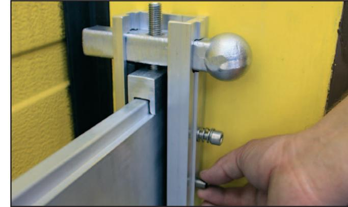
**8** On the front face of the demountable posts, by hand, start turning the 10mm cap head screws, clockwise, until they are finger tight.
