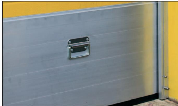
**2** Continue this process of inserting all flood boards along the entire barrier span, between each demountable post, until you reach the opposite vertical side channel.
