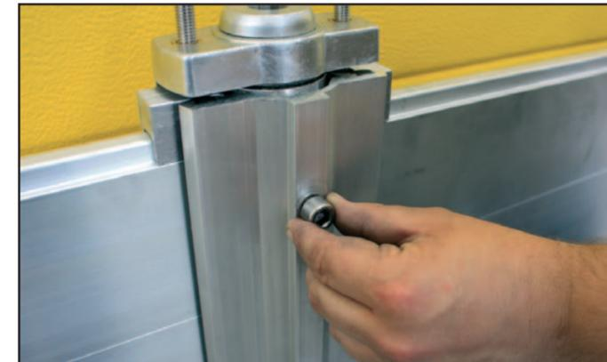
**9** Using the 5mm Allen Key, turn each grub screw and cap head screw, clockwise, one full turn (360 degrees)..
